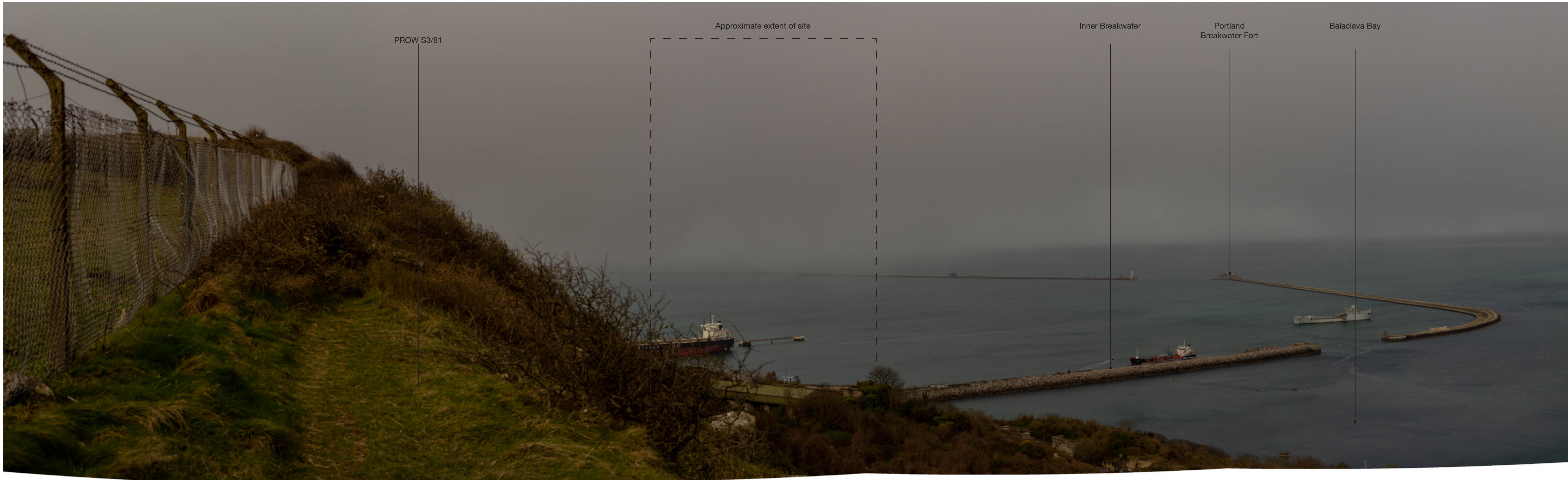
Taken from public right of way S3/81 Visualisation type 1. To be viewed at a comfortable arm's length and printed at A1
